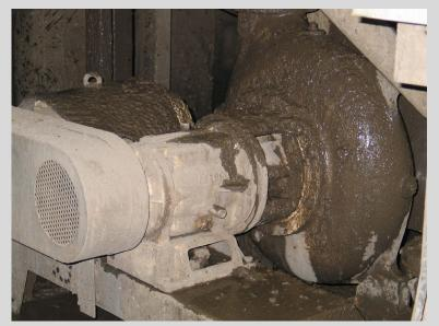
Significant contamination around this food processing pump challenged bearing life due to constant contamination ingress.
