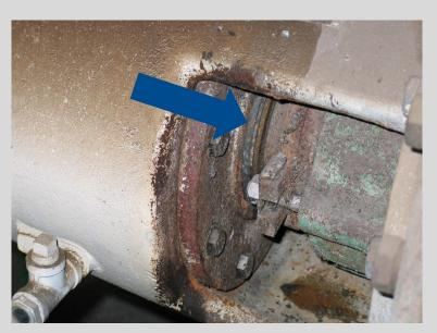
An installed Inpro/Seal Bearing Isolator in service for multiple years still performing with no issue.
